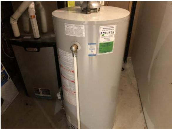
Photo 3: View of the typical hot water tank observed in all residential properties accessed on Site.
