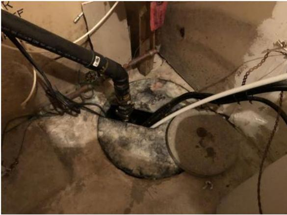
Photo 1: View of the typical sump pit and sump pump observed in all residential properties accessed on Site.
