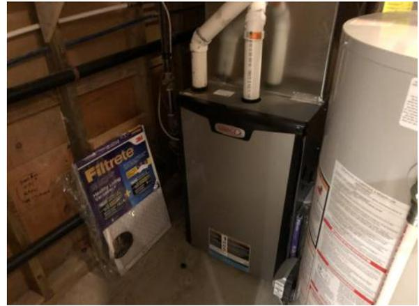
Photo 2: View of the typical natural gas fired furnace observed in all residential properties accessed on Site.
