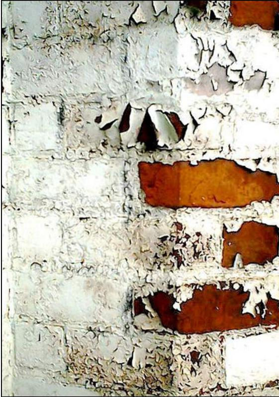
Non-breathing paint on brick. The vapour pressure of moisture in the brick blisters the paint, when it is able. If the paint adheres strongly, the pressure causes the brick surface to spall off, along with the paint, as seen in the centre of the picture. This lets in even more moisture, and the problem grows.
