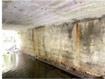
Wet Rusted Med to Severe Cracks on East Wall
