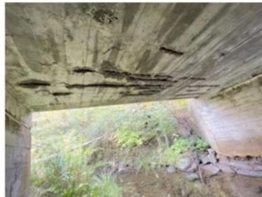
Soffit Excessive Severe Delamination & Exposed Rebars
